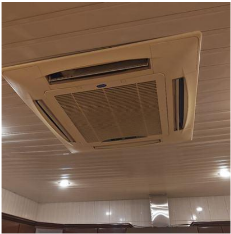
Kitchen - Air conditioner 10/05/2025 19:21
